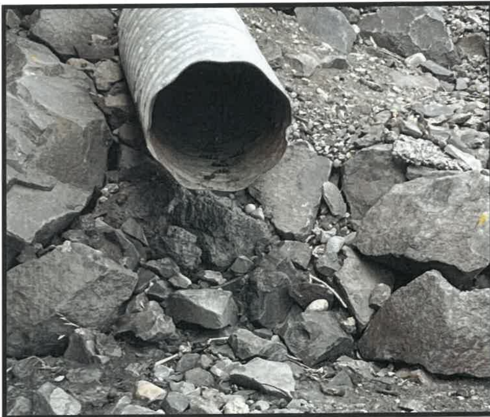
Figure 4: Stormwater outfall pipe in median with evidence of small mammal use.
