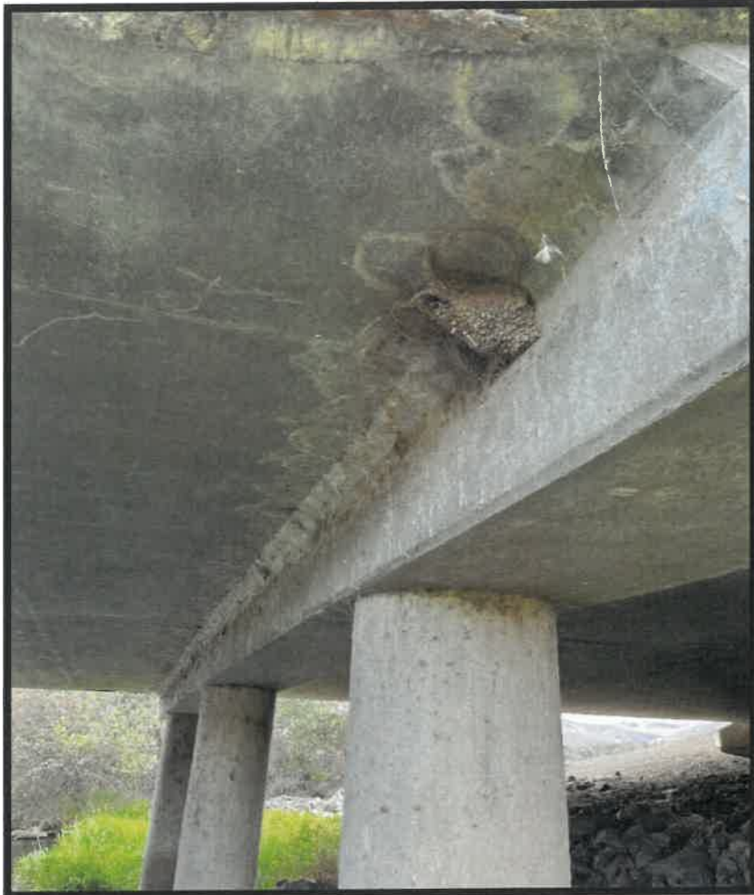
Figure 8: Inactive mud swallow nest beneath the WB Wilson Creek bridge.
