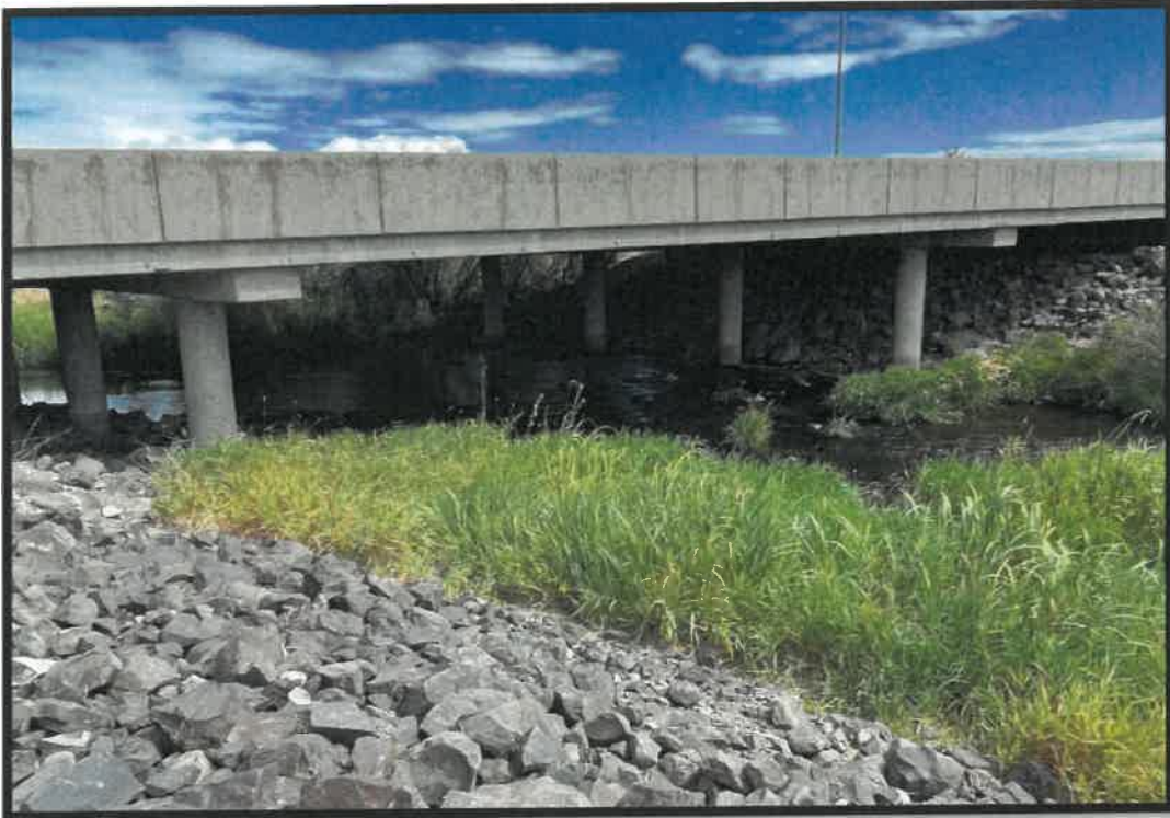
Figure 3: View of WB Wilson Creek Bridge facing northeast.
